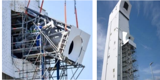
Centrifugal particle receiver
